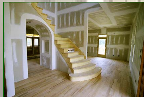
Residential Construction Final Clean
