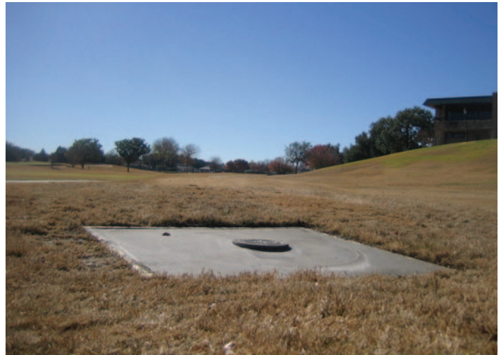
A piezometer pad is shown here in the Onion Creek golf course.
