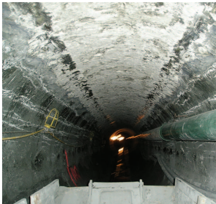
Underground tunnel will carry wastewater when completed (photo by Phillip Preslar).
