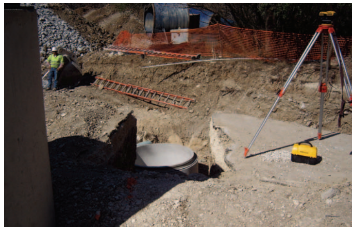
Manhole construction is underway.
