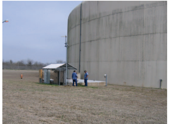
A pump station will be constructed at the Pilot Knob Reservoir site to provide water to current and future customers.
